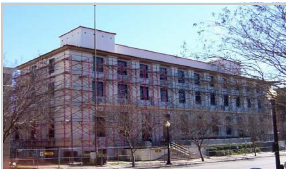
Upgrade/Renovate US Federal Courthouse Pensacola Florida
