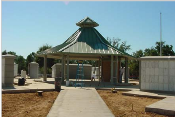
Construct Columbarium Complex Barrancas National Cemetery
