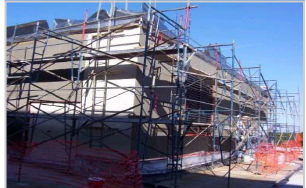
Renovation/Repair US Naval Hospital N.A.S. Pensacola
