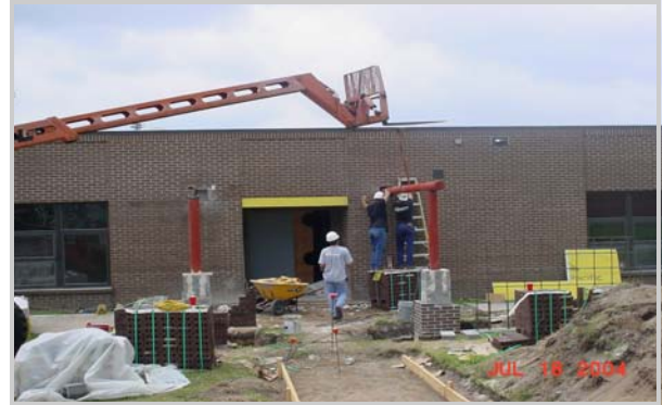
Classroom Addition Walton Middle School
