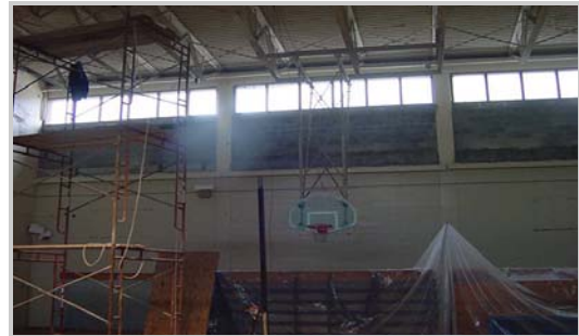
Renovate Fitness Center Eglin AFB, FL
